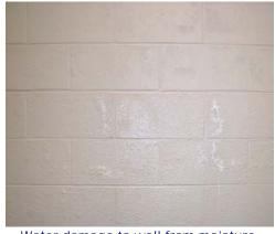
Water damage to wall from moisture penetration, Merrick Hall
